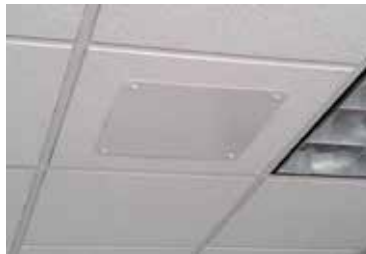
Installed Condition: PSIBVHF and PSIBVU78
